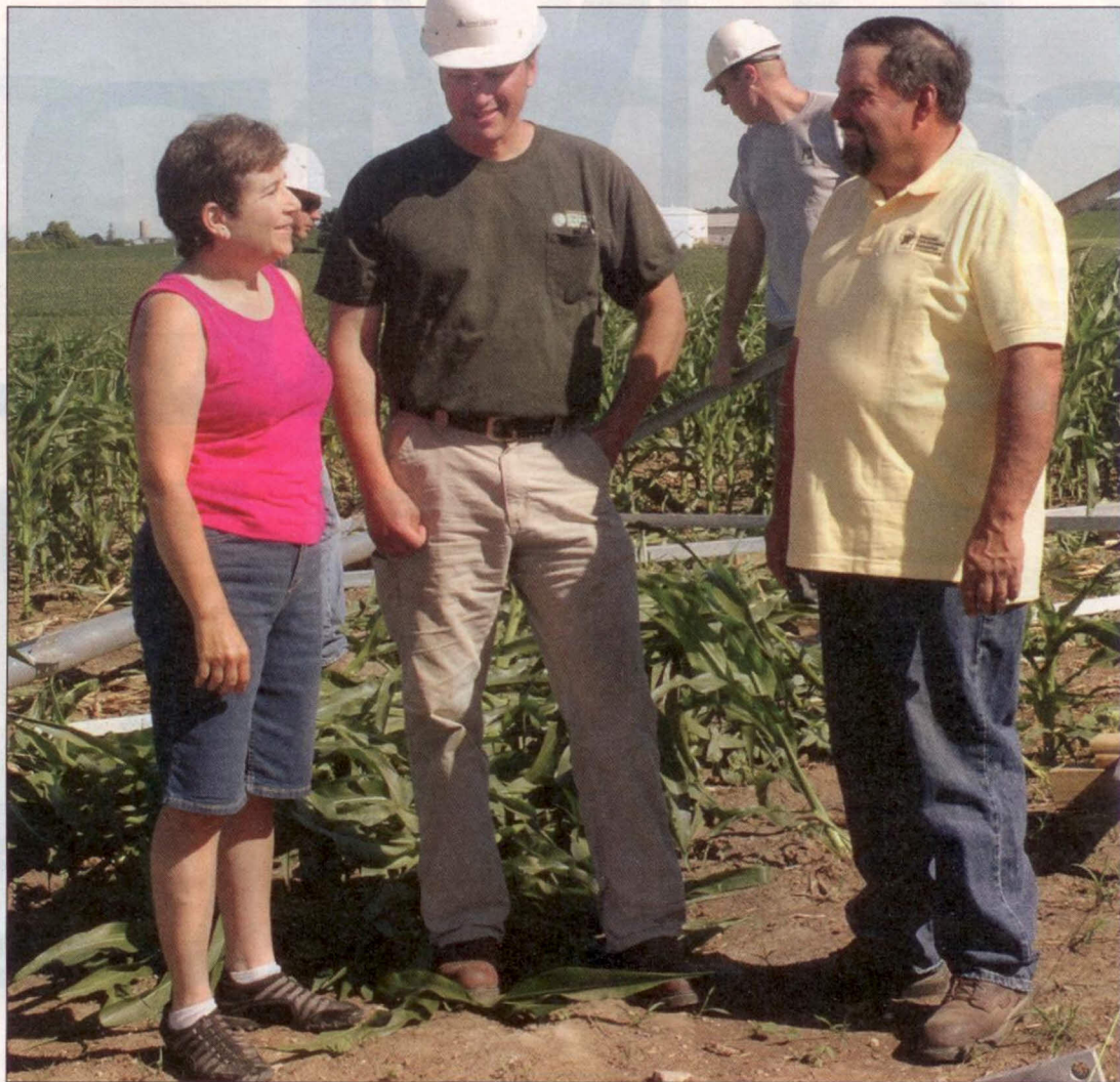
WIND ADVISER: Randy Faller (center) talks to Nancy Kavazanjian and Charles Hammer while workers begin erecting the wind turbine on the couple's farm.
